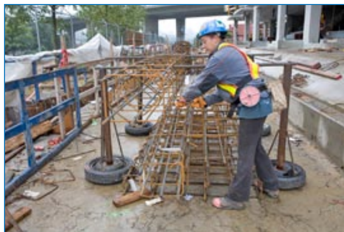
Prefabricate steel arrangements. This reduces forward bending.
