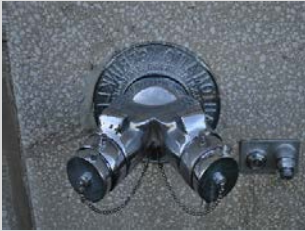
Fire Department Connection
