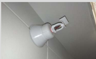
Sidewall Sprinkler
