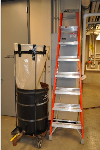
Do not block electrical panels.
