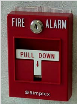
Fire Alarm Pull Station
