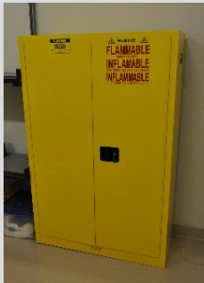
Flammable Storage Cabinet
