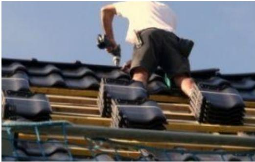
Photo Courtesy of ISHM: Workers MUST use fall protection when working on roofs.
